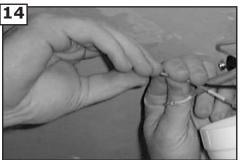
Make wire connections to power source using wire nuts provided. Make sure that no filiments are outside of the wirenut. After making the wire connections, the wires should be spread apart with the grounded conductor and the equipment-grounding conductor on one side of the outlet box and ungrounded conductor on the other side of the outlet box.
